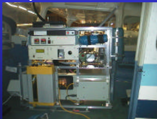
Port view of rack
